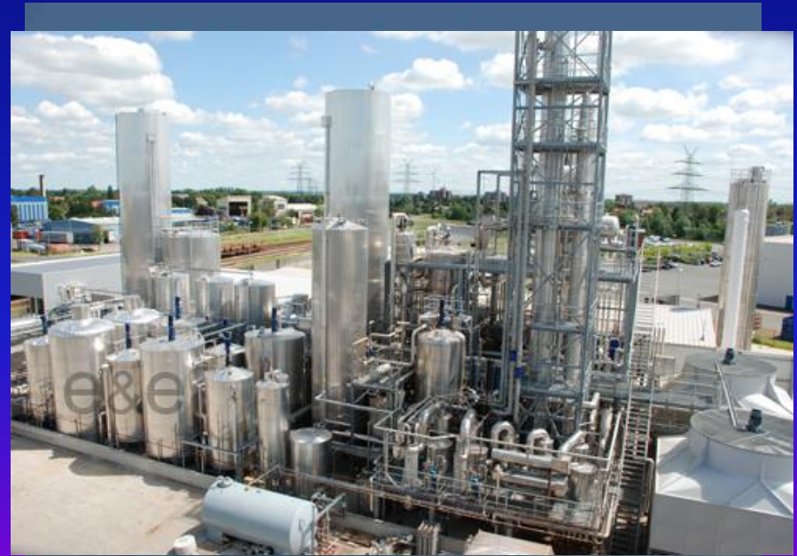
Seawater distillation plant
